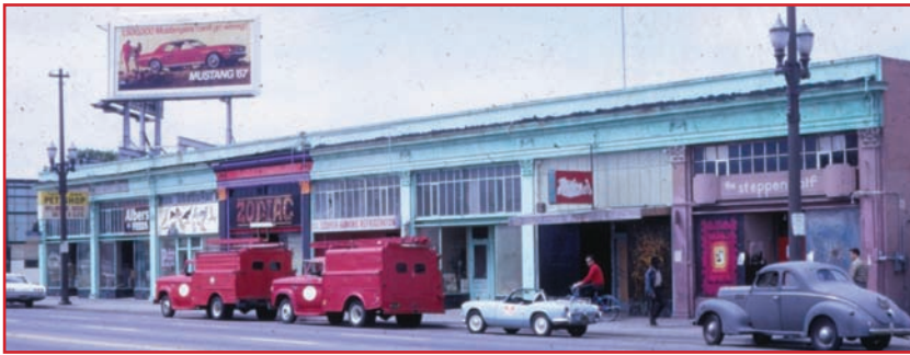
The Borg Building in 1967 (Humphrey slide collection, BAHA archives)
