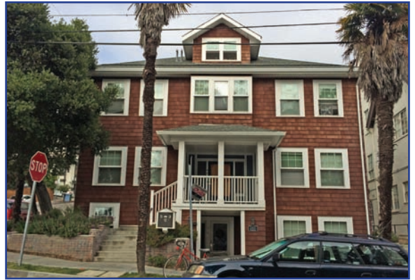
The rebuilt house in July 2019. Anthony Bruce.
