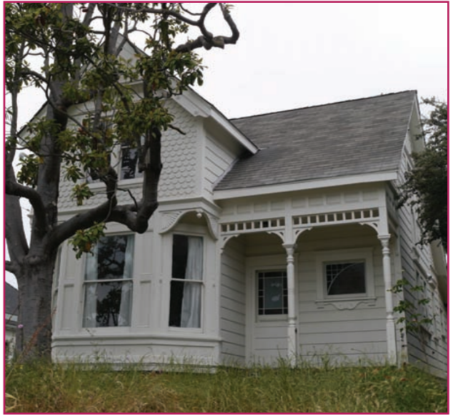
The house at 1731 Addison Street with overgrowth cleared and a new coat of paint. James Angus, 2019.
