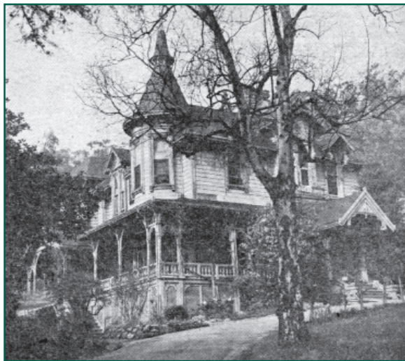
The Garber House as it looked shortly before it was demolished. Berkeley Daily Gazette photo, 1958.
