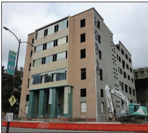
Demolition of 2223 Fulton Street underway. Steven Finacom, March 2019.
