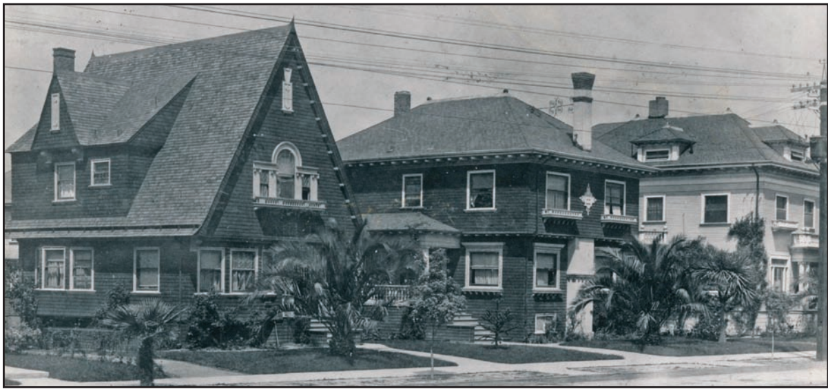
A typical group of J. A. Marshall speculative houses designed by C. M. Cook. These were built on Telegraph near Derby in late 1904. Marshall family photo, BAHA Archives.
