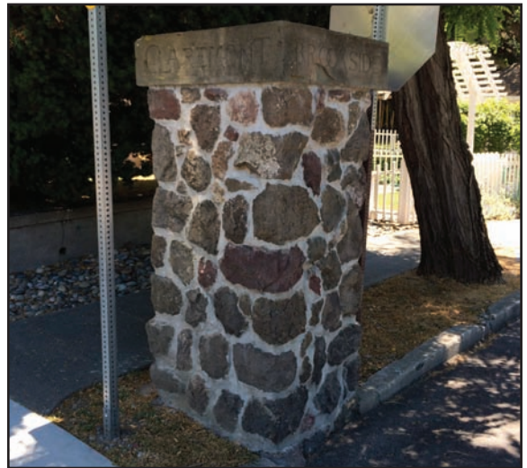
Reconstructed pillar at Brookside. Anthony Bruce, 2017.
