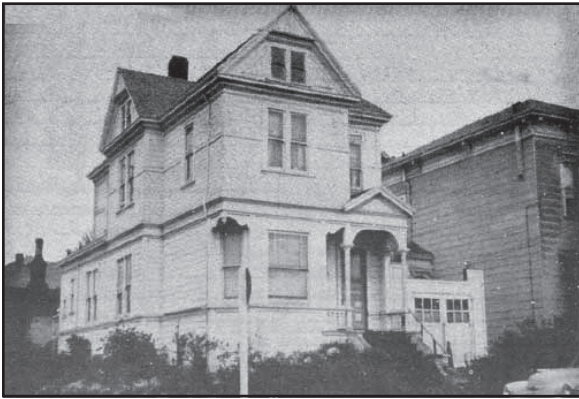
The Clark House of 1878, at 2005 Berkeley Way, seen at the right in this 1955 photo. Donogh File, BAHA Archives.
