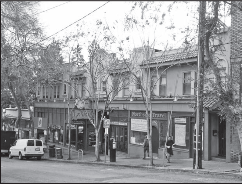
The 1800 block of Euclid Avenue; historic mixed-use districts could be at risk. Daniella Thompson photo.
