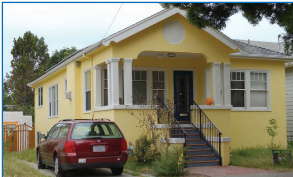
The Felt House on Jefferson Ave. Carrie Olson, 2015.
