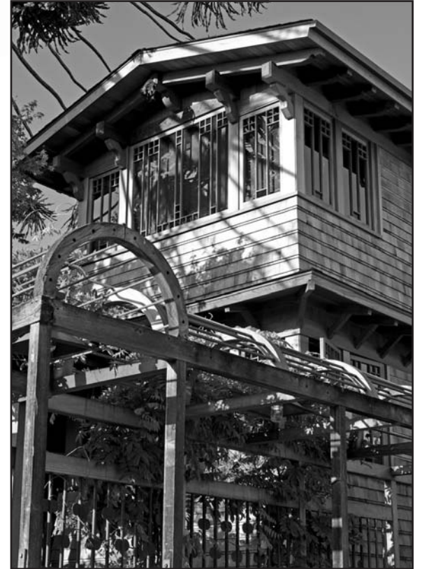
Chez Panisse. Rebuilt porch and trellis. Carrie Olson, 2014.
