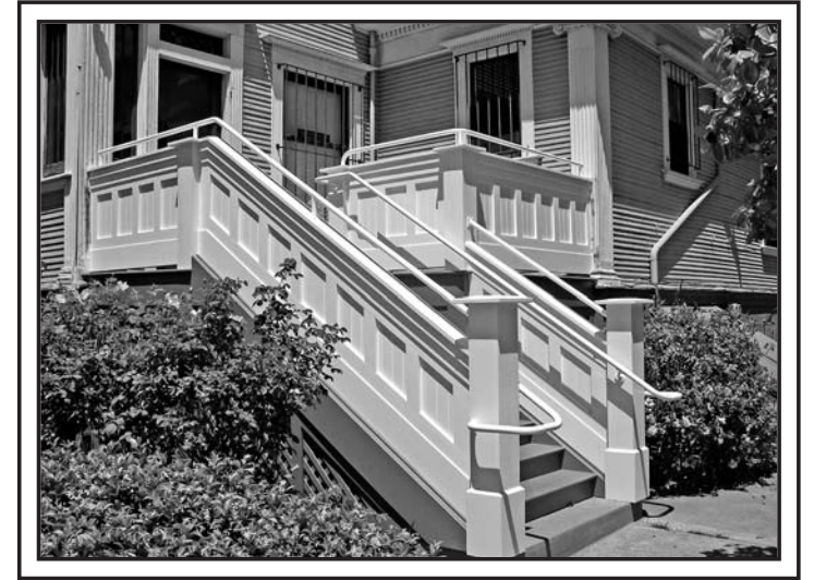
The newly completed entry porch to the BAHA office. John McBride, 2014.
