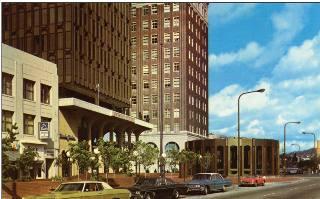
This Mike Roberts postcard from the 1970s, published by the Berkeley Chamber of Commerce, is entitled "BART Station, Downtown Shattuck Avenue." It shows the newly completed BART rotunda on Shattuck at Center, an especially prominent above-ground structure in the BART system: not merely a slit in the sidewalk for either stairs and/or an escalator, in and out of the system.
