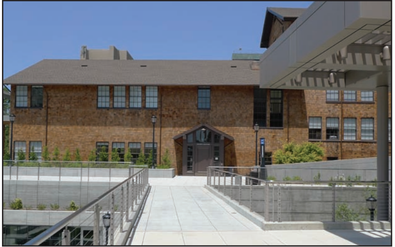
View of Naval Architecture Building from the south. Carrie Olson, 2011.
