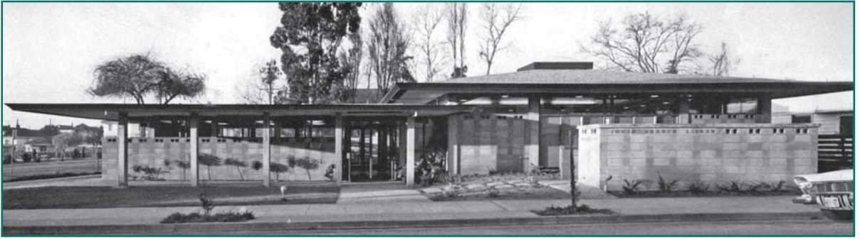
The South Berkeley Library (John Hans Oswald, Architect, 1960). Karl H. Riek, photographer, from John Hans Oswald, Architect (Donald Reay and Peter Paret, 1975).
