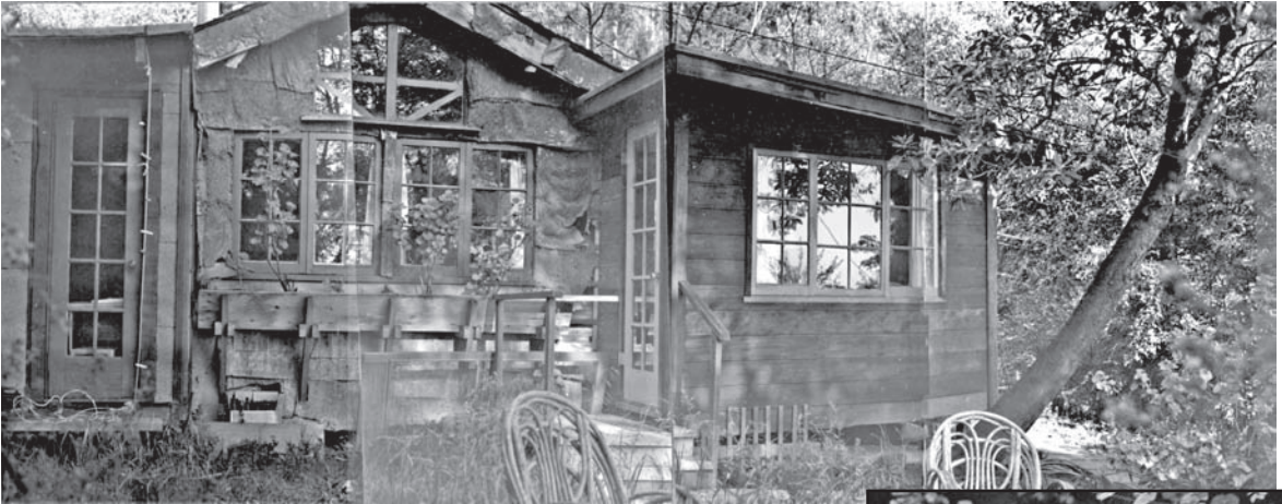
The west side of the Cottage showing the 1957 addition to the right and two pieces of willow garden furniture in the foreground. Photo c. 1959, BAHA Archives, gift of Katherine Trow.
