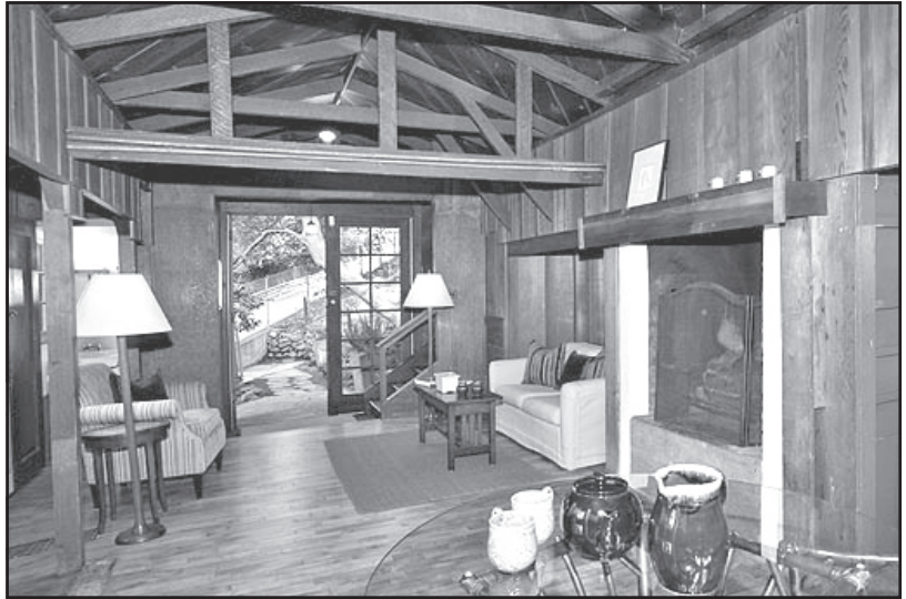
The long, narrow main room of the Cubby House reflects its original use as a home for a large Packard. Note the exposed trusswork, with rafters stained blue-green. To the right is a concrete “Maybeck” fireplace, built to a smaller scale than is typical. Liz Rusby photo, courtesy The Grubb Company.
