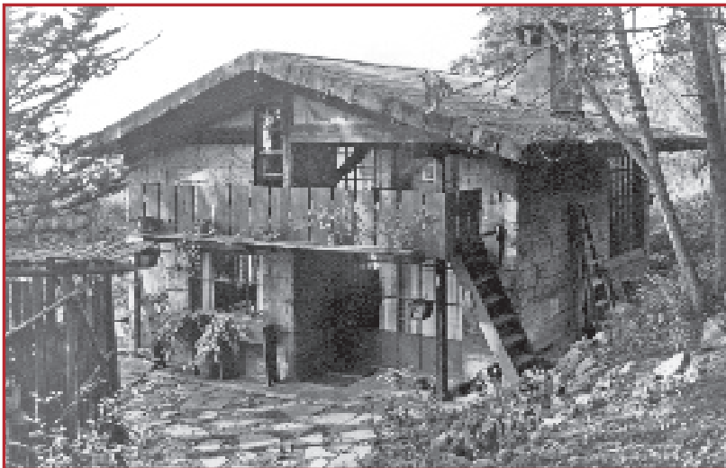
A side view of the Maybeck Studio (1924), its walls sheathed in burlap sacks dipped in Bubblestone. Lionel Berryhill photo, Dimitri Shipounoff Collection, BAHA Archives.
