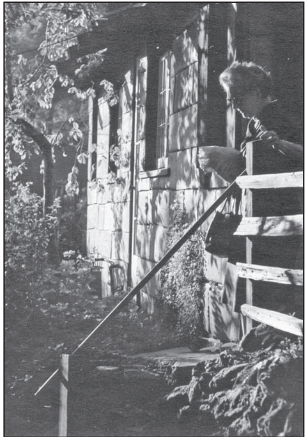
Mamie Minor at the door of the Cubby House. This view clearly shows the Bubblestone siding. Courtesy of the Minor Family.
