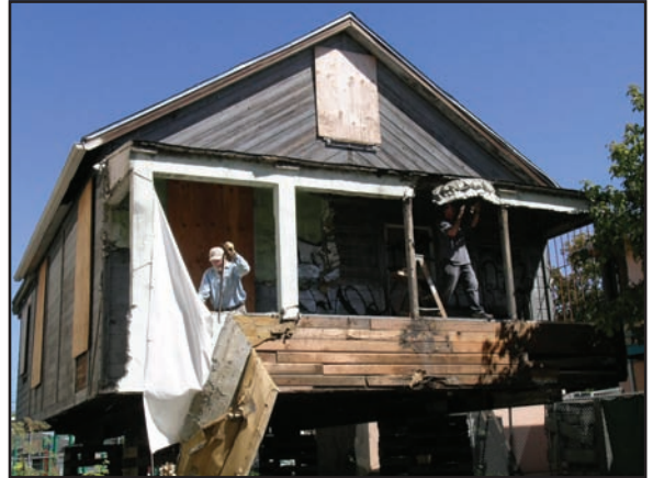
The first step in restoring the Kenney Cottage to its original appearance was to remove the stucco covering its board walls. Richard Ehrenberger and Richard Wesell are shown here at a BAHA work party in the process of exposing original redwood boards. Daniella Thompson, 2004.
