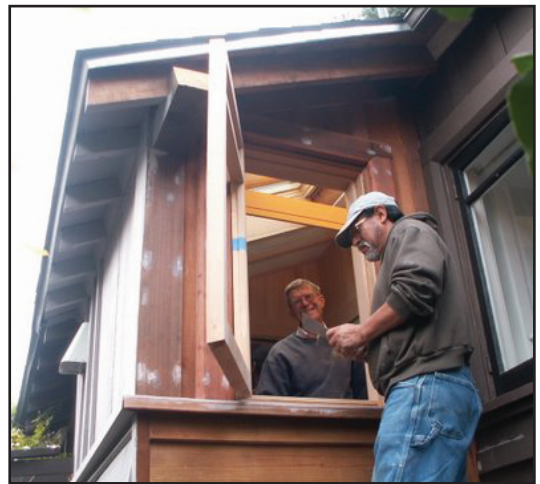
Grant Street addition under construction. Jacqueline Beth.
