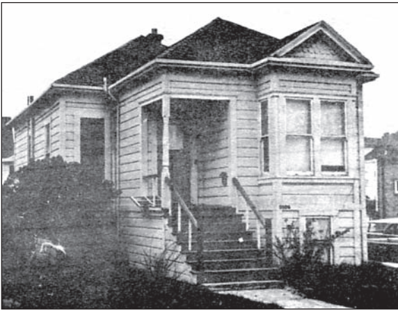
This one-story Queen Anne Cottage above a half-story raised basement is typical of a working man's house, placed on a small "urban" rectangular lot, that was once prolific in Victorian Era neighborhoods in the East Bay. It has a projecting front bay, high cut-away recessed porch, and no single roof line under oversized gables. 1964 image, Donogh File, BAHA Archives.
