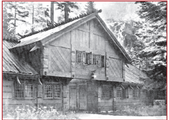
View of the Caretaker’s House at Vikingsholm from courtyard. Note spiked wooden gutter construction that is described here.
