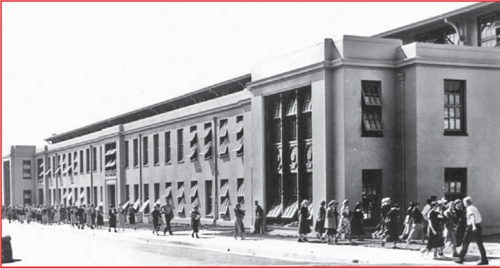
The Berkeley High School Gymnasium as it appeared after the 1937 seismic work by Thomas Chace—and as it looks today. BAHA Archives.
