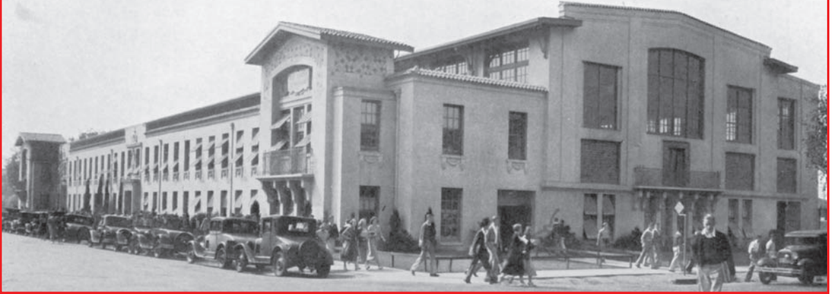
The Berkeley High School Gymnasium (William C. Hays, 1922) as it appeared after major additions designed by Walter H. Ratcliff, Jr., in 1929. To the left is the long Milvia Street frontage that is still a handsome presence. December 1932 Olla Podrida.
