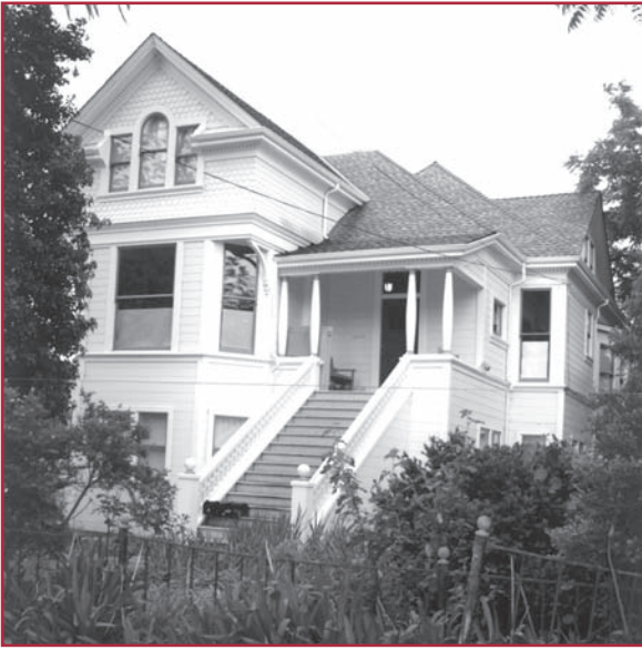
The restored Hunter House with its new staircase. Carrie Olson, 2006.
