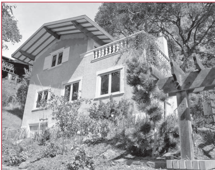
The Jockers House after restoration. Daniella Thompson, 2006.
