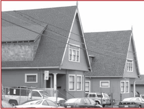
High-Peaked Colonial Revival houses at 2132 and 2130 Haste Street, designed by C. M. Cook in 1905. Daniella Thompson, 2005.
