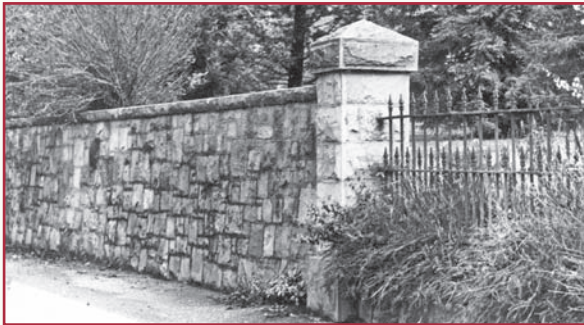
A section of the wall along Warring Street. Anthony Bruce, 1979
