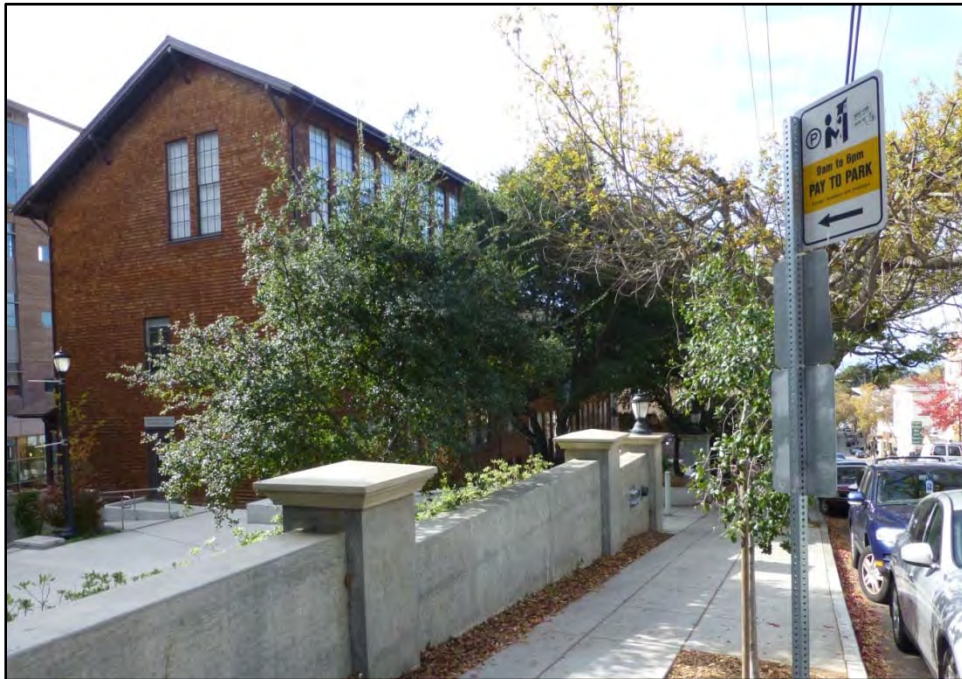
Photograph 2. Naval Architecture/Blum Hall (NRHP 76000475) shown at left; facing west, November 12, 2014.
