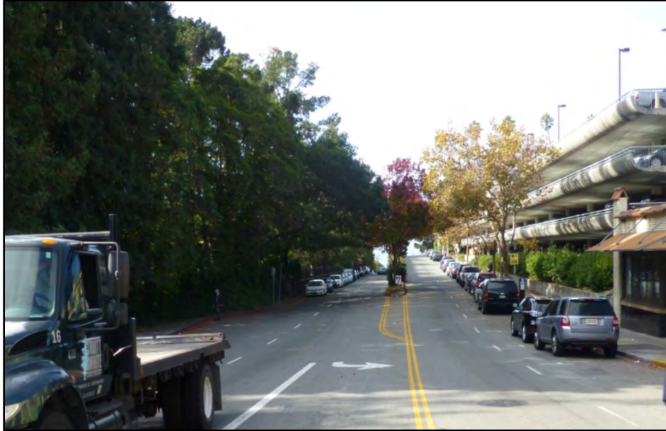
Photograph 5. Hearst Avenue showing split in the road; facing West, November 12, 2014.
