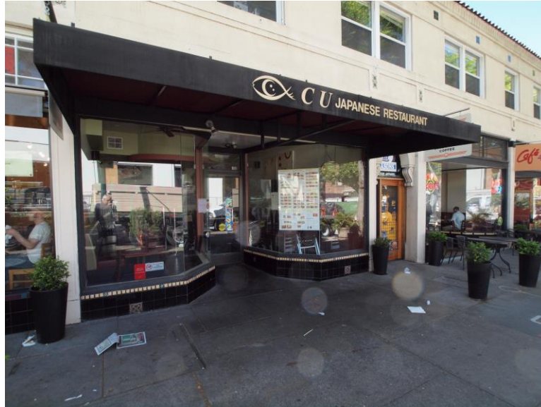
Typical storefront, viewed facing southwest.
