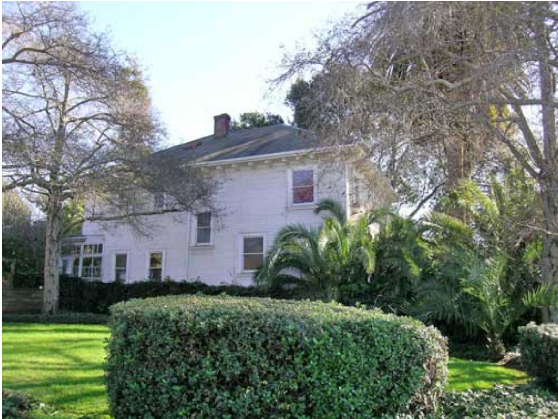
Figure 16. North façade, seen from the Hearst-MLK corner
