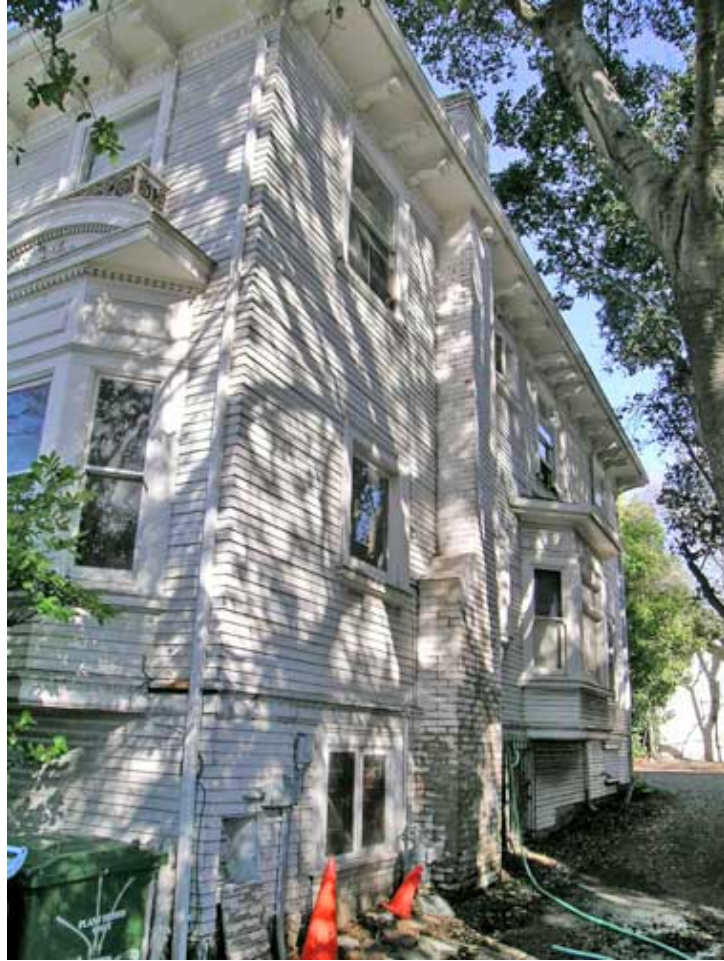
Figure 17. South façade, looking east
