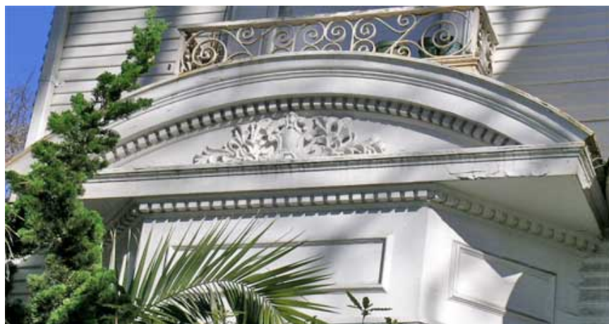
Figure 12. Pediment & cornice above window bay, west façade
