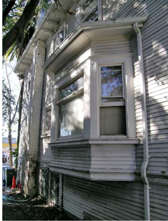
Figure 21. Window bay, south façade
