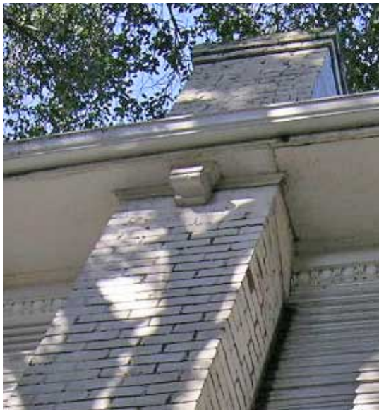
Figure 18. Left: corbel head on chimney. Right: corbel profiles on south façade
