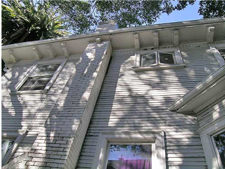
Figure 19. South façade, front part
