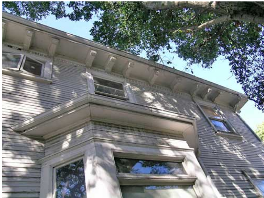
Figure 20. South façade, rear part
