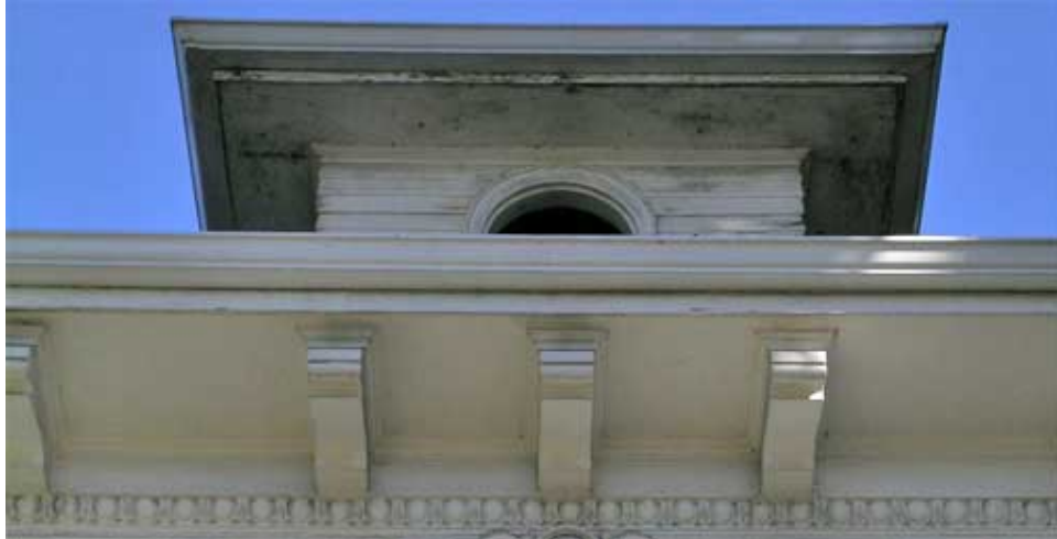
Figure 8. Roof eaves & cornice ornaments
