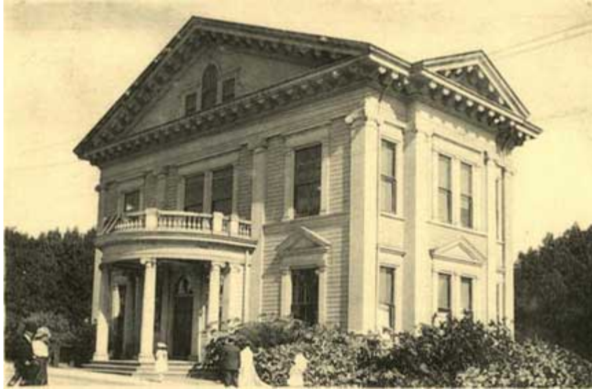
Figure 47. The first Botany Building at U.C. Berkeley
