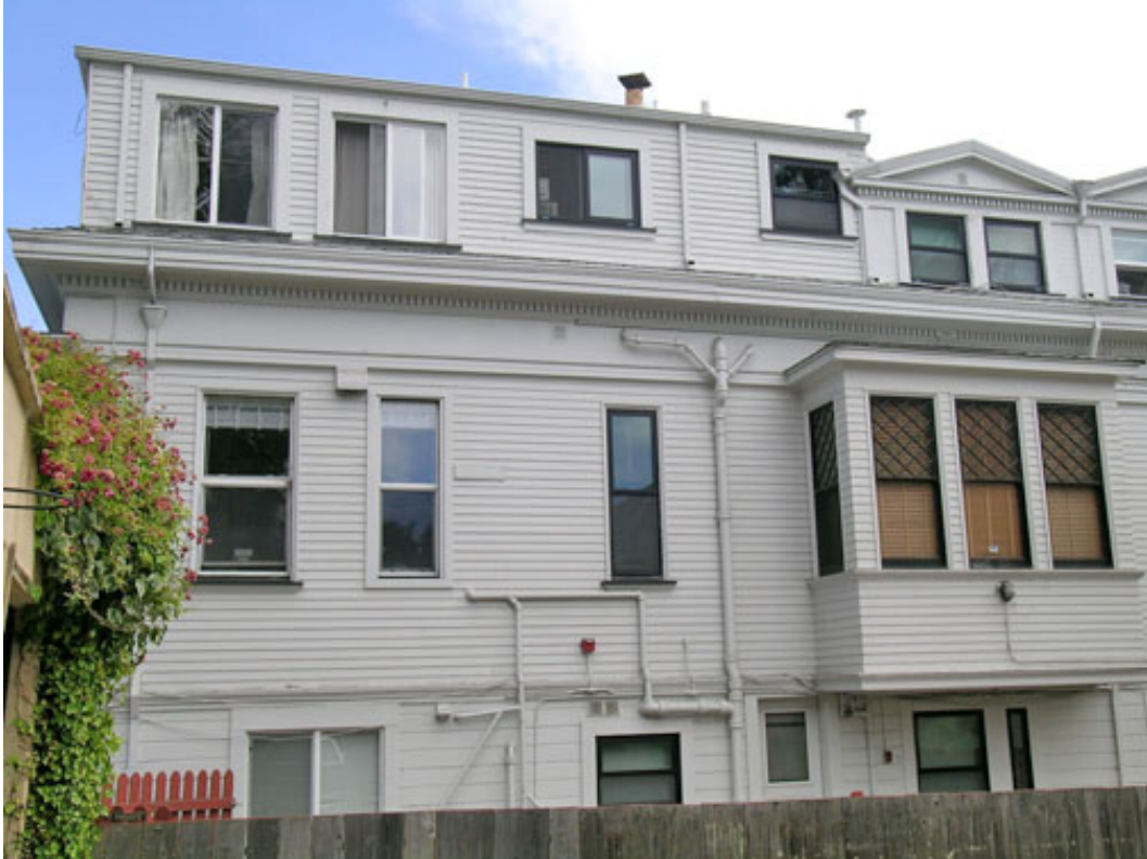
Figure 33. North façade, eastern part
