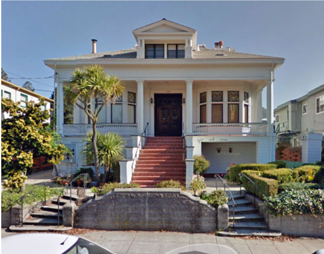
Figure 18. Street façade (Google Street View, Jan. 2015)
