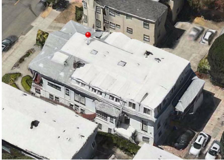
Figure 38. South façade (Apple Maps)
