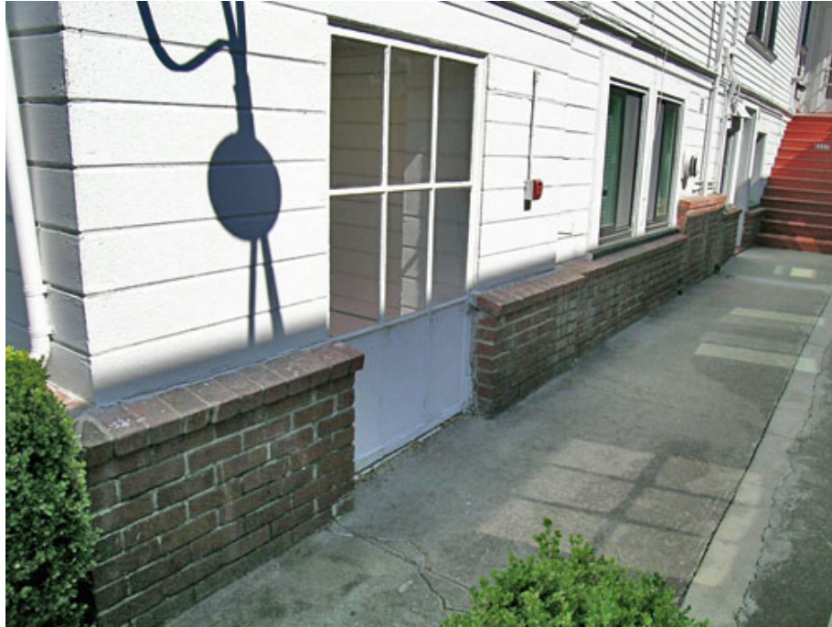
Figure 47. Ground floor, south façade
