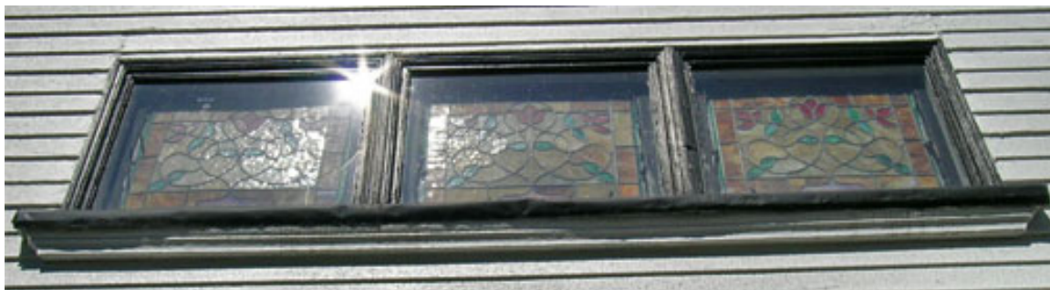
Figure 41. Horizontal window at west end of south façade
