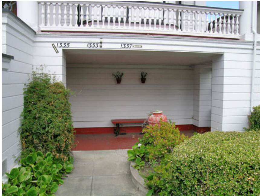
Figure 26. Ground-floor recessed lobby to basement apartments
