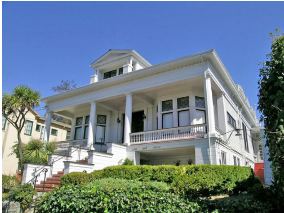
Figure 2. Captain Slater House, September 2016 (photo: Daniella Thompson)
