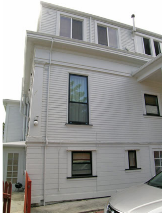
Figure 51. Corner pilaster, east façade
