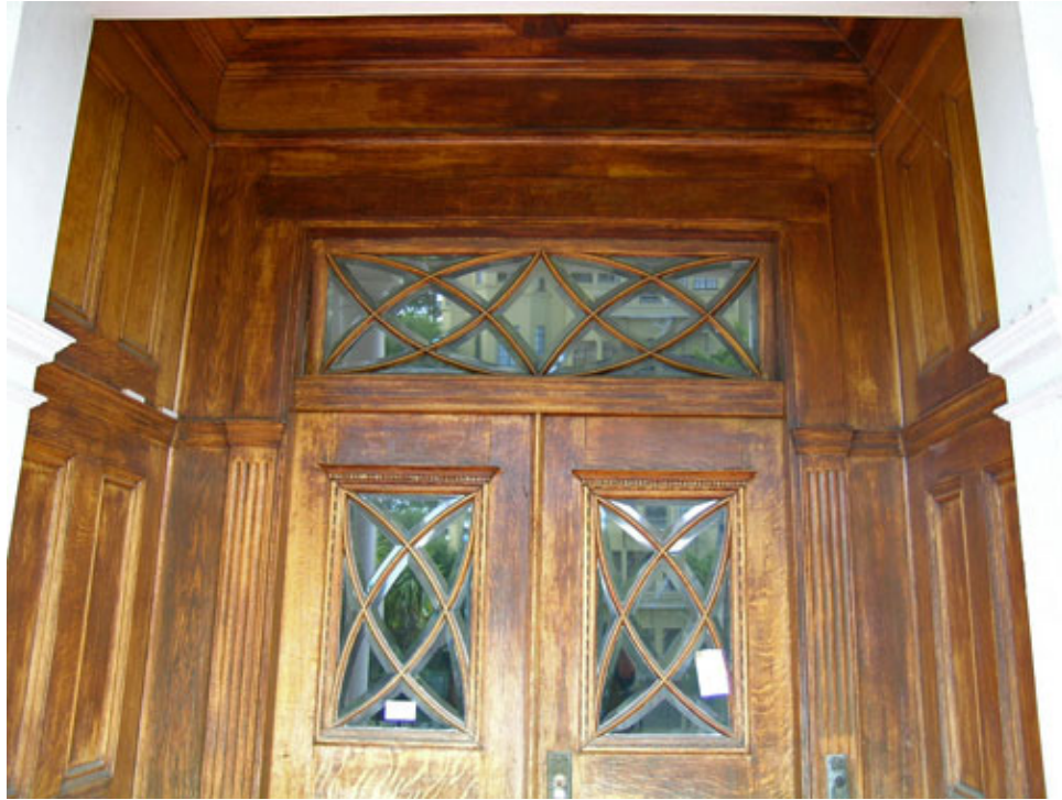
Figure 24. Front door niche
