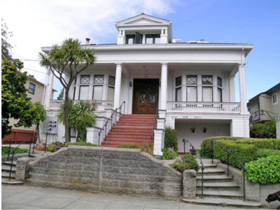
Figure 5. Street façade and retaining wall
