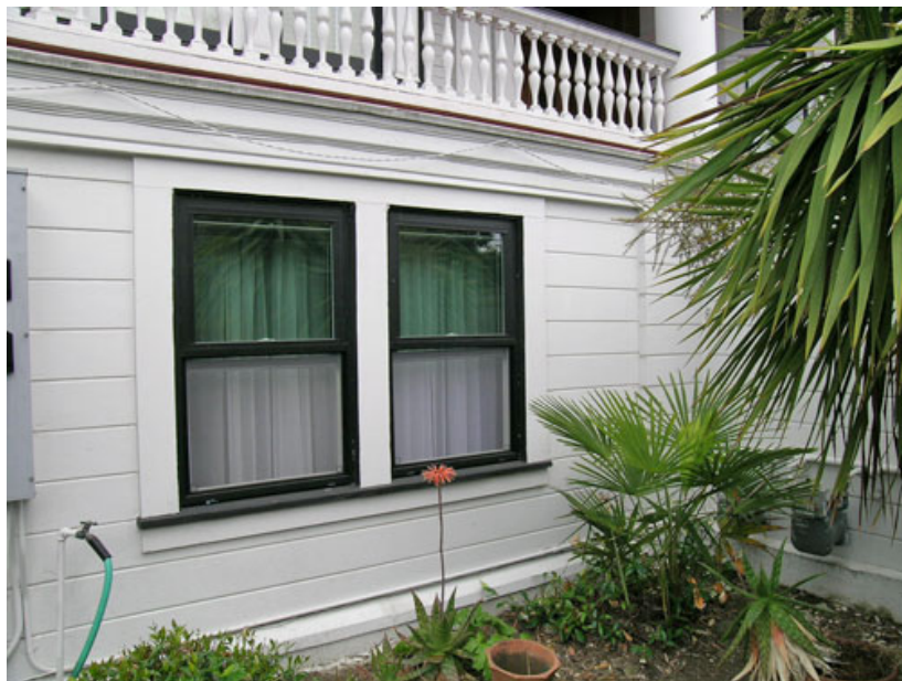
Figure 29. Double-hung windows under porch
