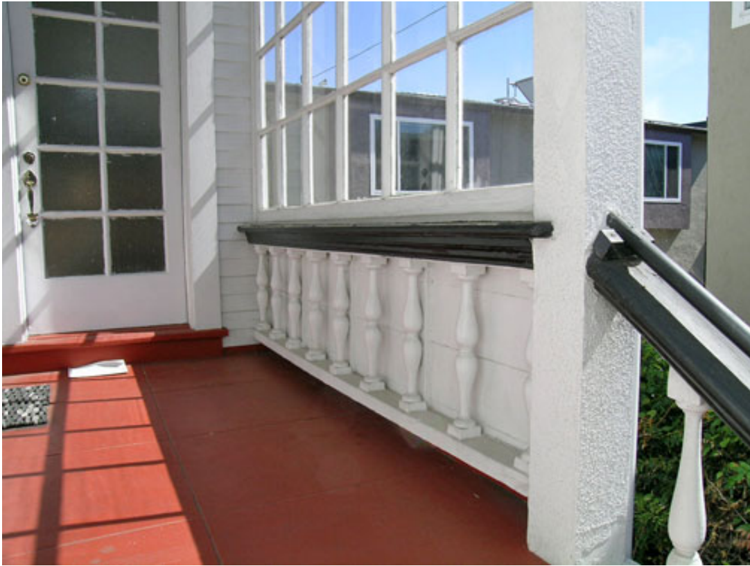
Figure 45. South porch interior
