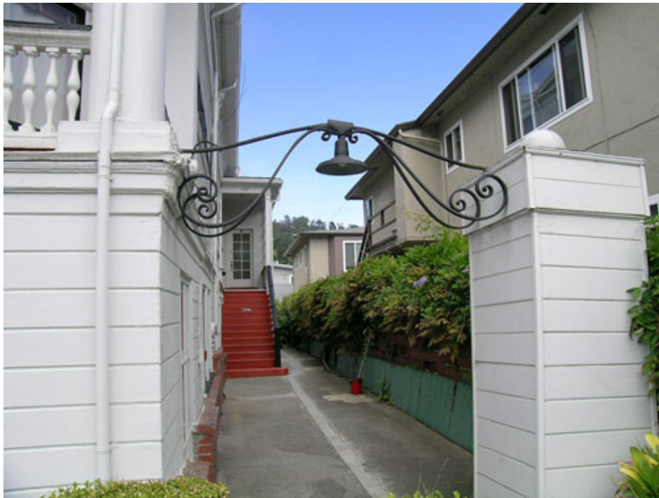
Figure 39. Gateway to south side
