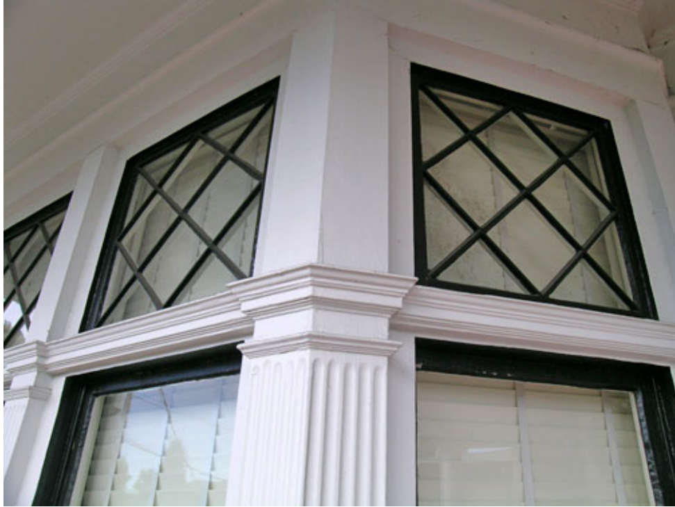
Figure 22. Bay window & pilaster detail
