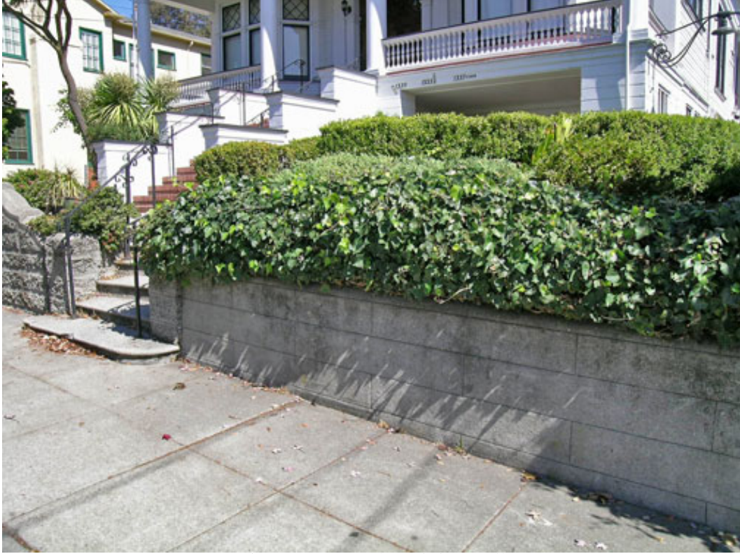
Figure 13. Scored retaining wall
