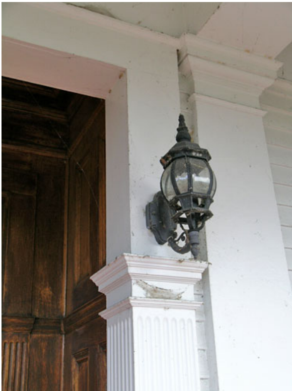
Figure 25. Doorway pilaster & capital
