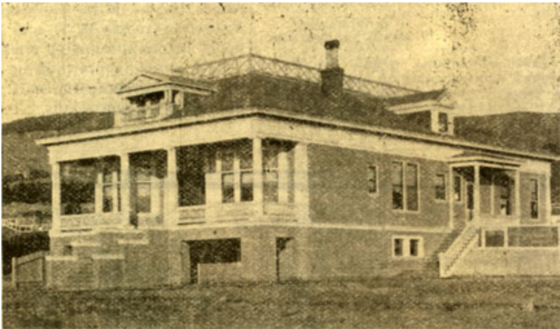
Figure 6. The Slater House as depicted in the Berkeley Herald, 1 January 1896
