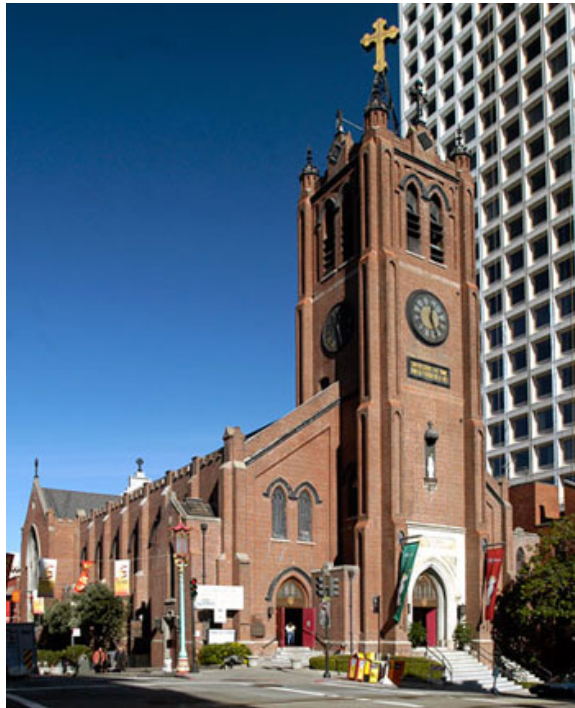
Figure 92. Old St. Mary's Cathedral ( Noehill )
