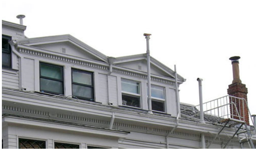
Figure 34. Dormers & chimney, north façade
