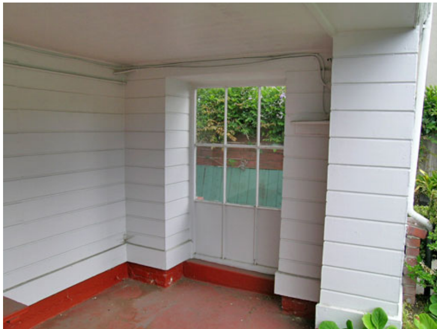
Figure 27. Fixed window in ground-floor open lobby
