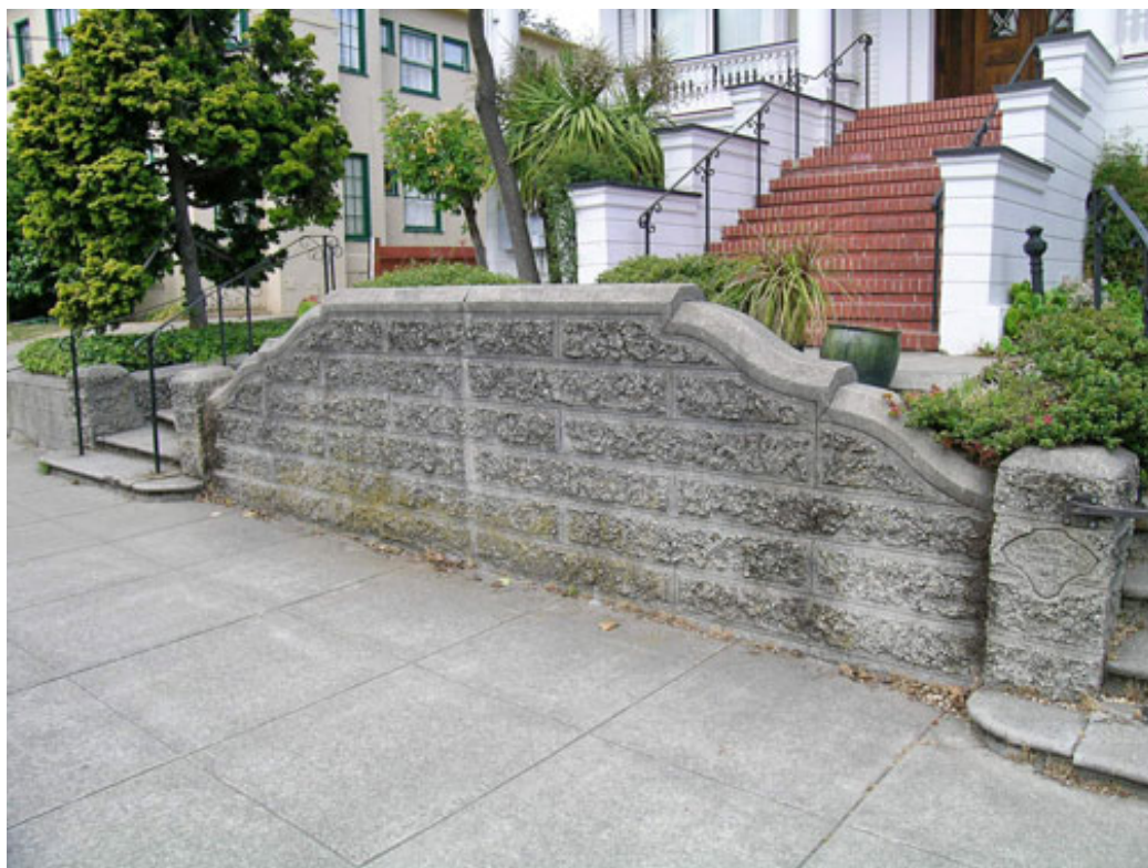
Figure 9. Rusticated concrete retaining wall built by John A. Marshall
