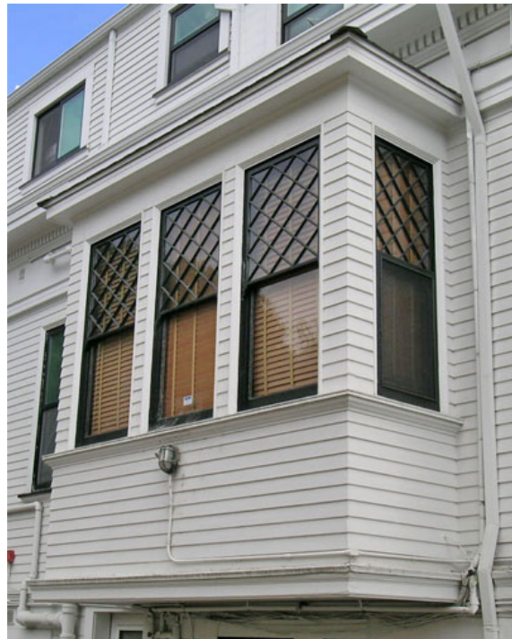
Figure 35. Boxed window, north façade
