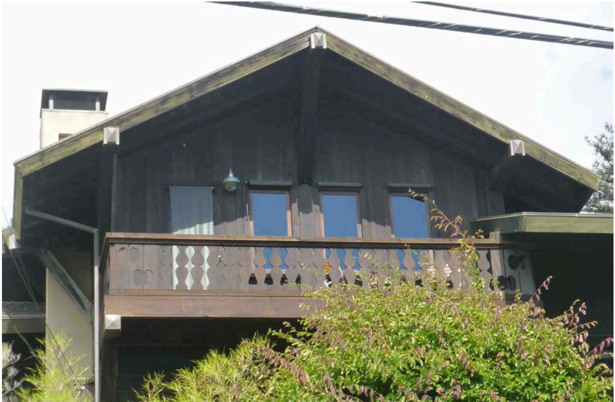
(Above. Top floor of west facade, top floor balcony under gable. Note metal caps on ends of roof supports, Venturi form chimney top at left, and canted southwest corner roof form at right. Below, detail of southwest roof corner. At left. View of basement level of west elevation, looking southeast towards entry path. New patio outside basement in foreground. (Photo S. Finacom, 2021.)
