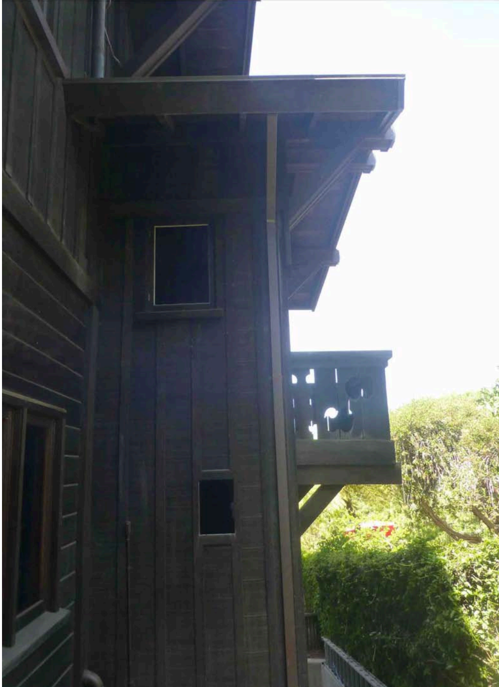
(At left, looking west, along the north wall of the original house, showing the one and a half story board and batten bay that contains the stairwell. The “Juliet” balcony is on the right, and there is a small hipped roof over the projecting bay. Photo S. Finacom, 2021.)
