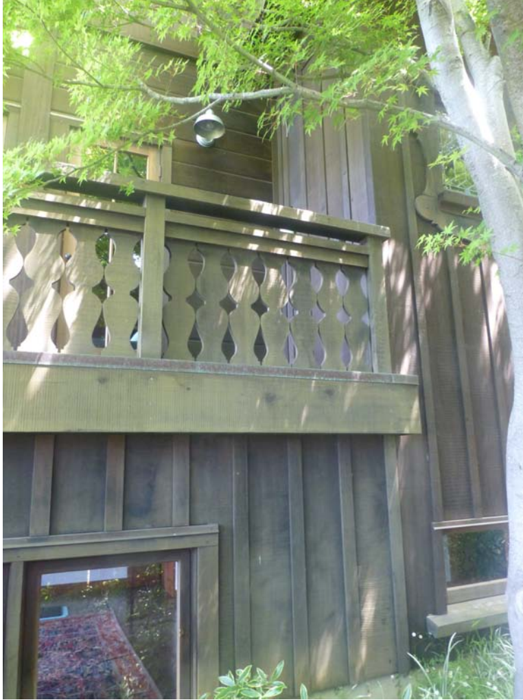
(At left. View of south wall, showing lower balcony and how it dead-ends into vestibule wall; one of the French doors to balcony from living room; change in siding from horizontal boards to vertical boards and battens at main level. Photo S. Finacom, 2021.)
