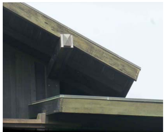
(Above. Top floor of west facade, top floor balcony under gable. Note metal caps on ends of roof supports, Venturi form chimney top at left, and canted southwest corner roof form at right. Below, detail of southwest roof corner. At left. View of basement level of west elevation, looking southeast towards entry path. New patio outside basement in foreground. (Photo S. Finacom, 2021.)
